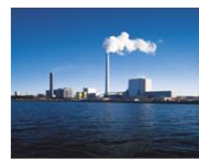
Biomass steam Kal (2019)
